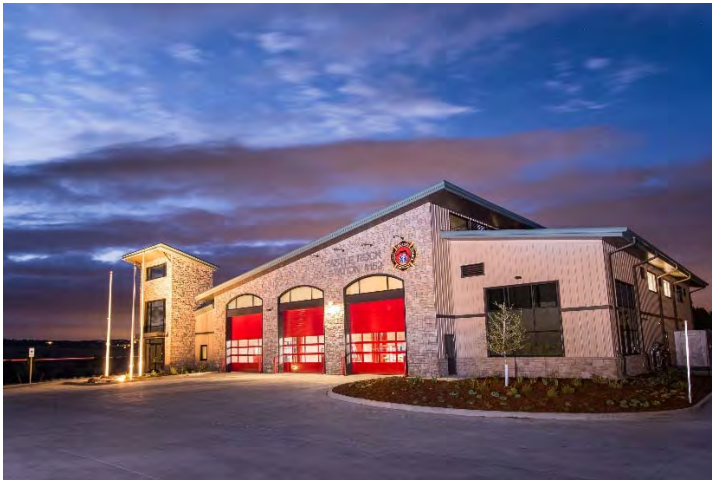
Fire Station 152 opened in the Crystal Valley area of Town; 12 positions were added to staff the station.
